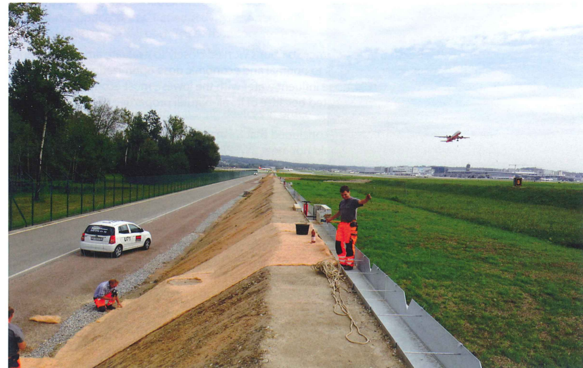
Installation of wood wool at the Zurich airport.
