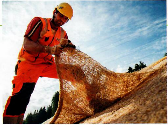
Wood wool fleeces provide erosion control on slopes and can help protect seedlings from temperature fluctuations and dry periods.
