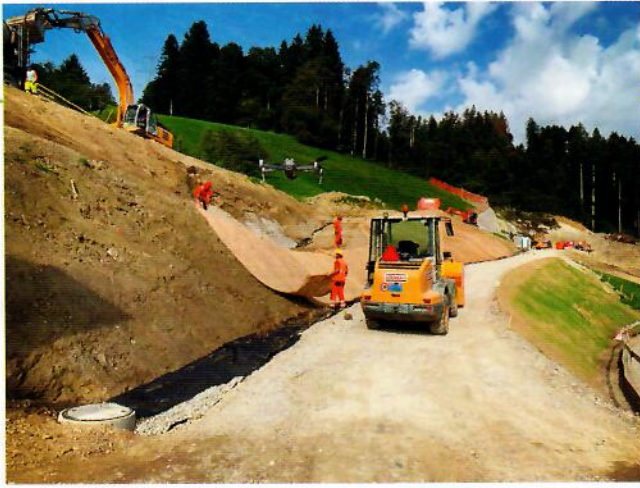
Wood wool fleeces provide erosion control on slopes and can help protect seedlings from temperature fluctuations and dry periods.
